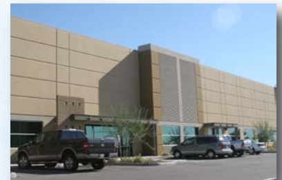
WEST & EAST COAST FACILITIES (AZ SHOWN)
